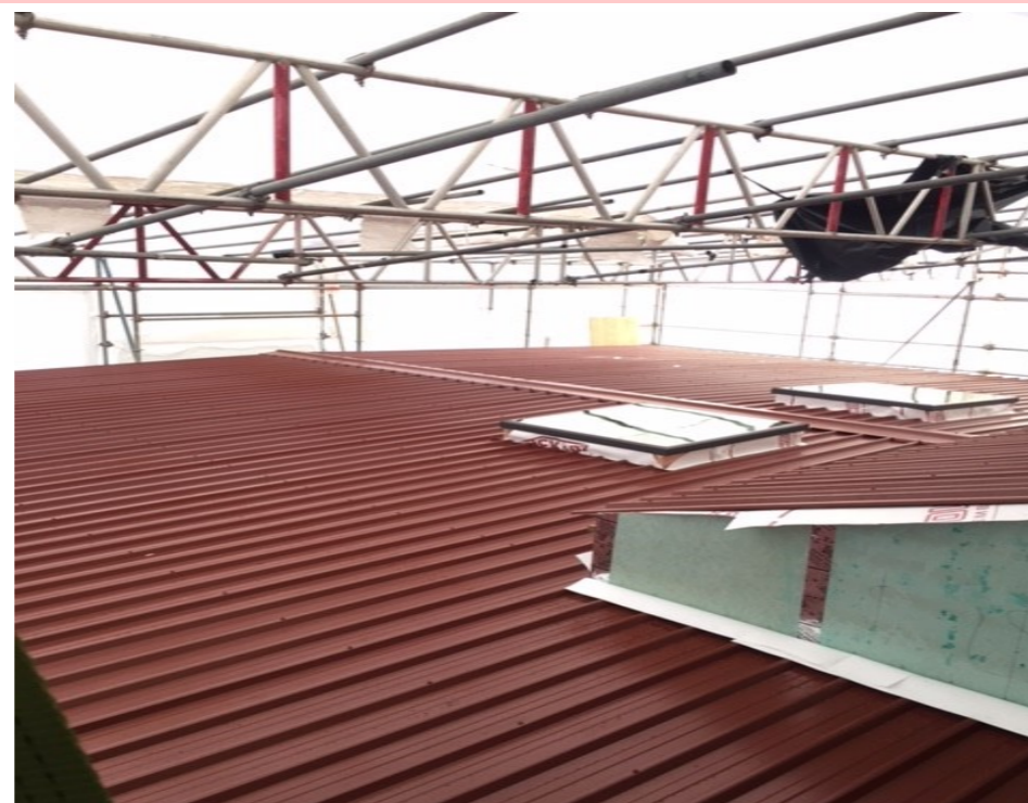
A NEW ROOF ON C BLOCK!
